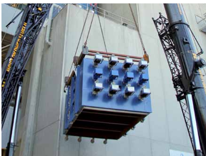
Installation of waste heat recovery boiler at Finnish cement company Finnsementti Oy.
